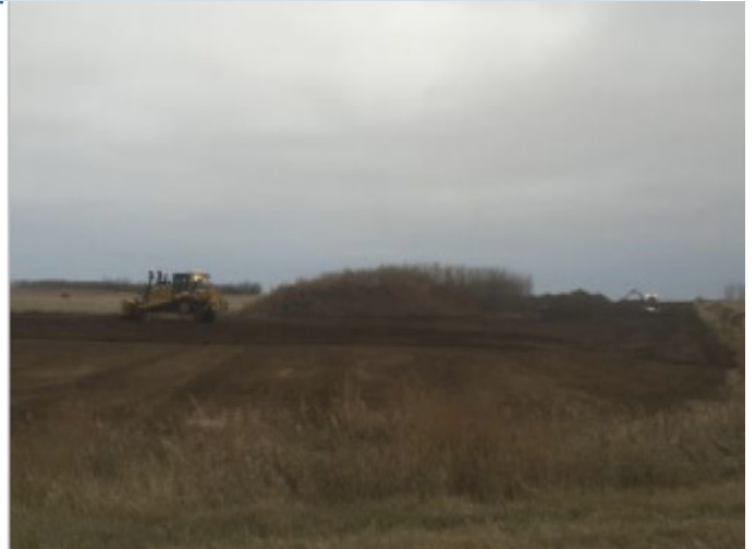
Dozer spreading out seconds – SF 34 – Oct 11, 2018
