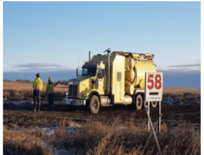
Crew at ovality dig site – SF 58 – Oct 13, 2018
