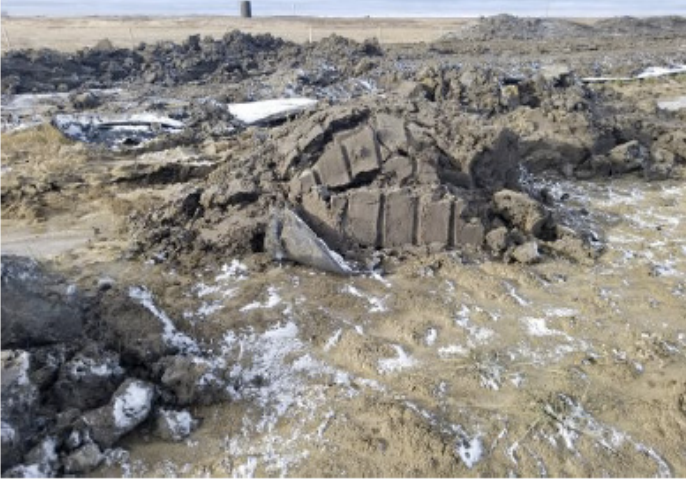
Buried geotec wetland ramp material - SF 39 - Oct 13, 2018
