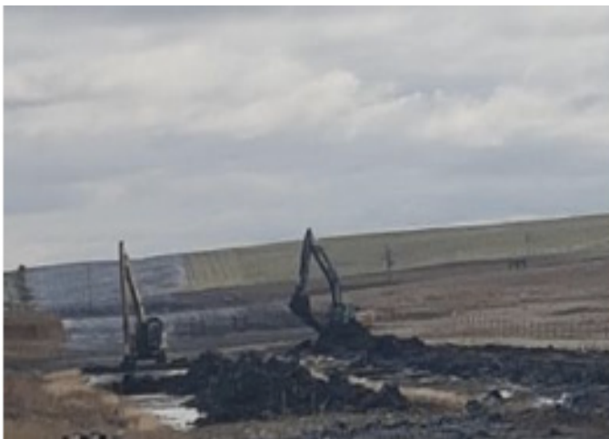
Excavators working on wetland removing geotec– Km 62+600 -Oct 13, 2018
