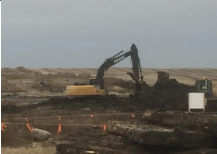
Wetland ramp removal – SF 44 – Oct 11, 2018
