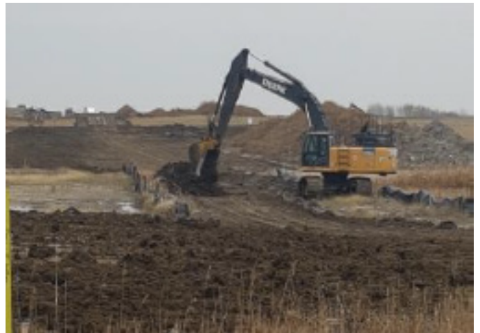
Excavator working on wetland ramp removal – SF 46 – Oct 11, 2018
