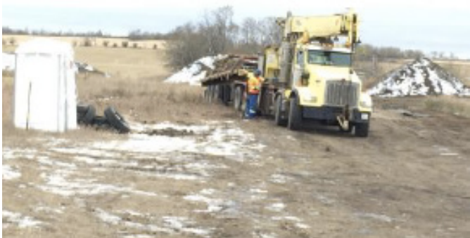
Rig mat removal – SF 25 – Oct 10, 2018
