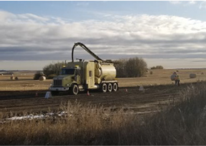
Hydro-vac day lighting pipe – SF 53 – Oct 10, 2018
