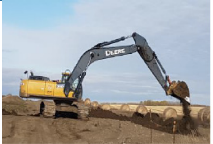
Excavator working on grade – SF 58 – Oct 10, 2018
