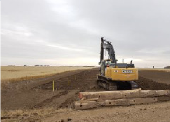
Dig site staked and ready - SF 86 - Oct 12, 2018
