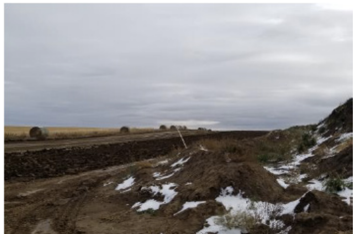
Surveyors staking anomalies from pig test– SF 53 -Oct 9, 2018
