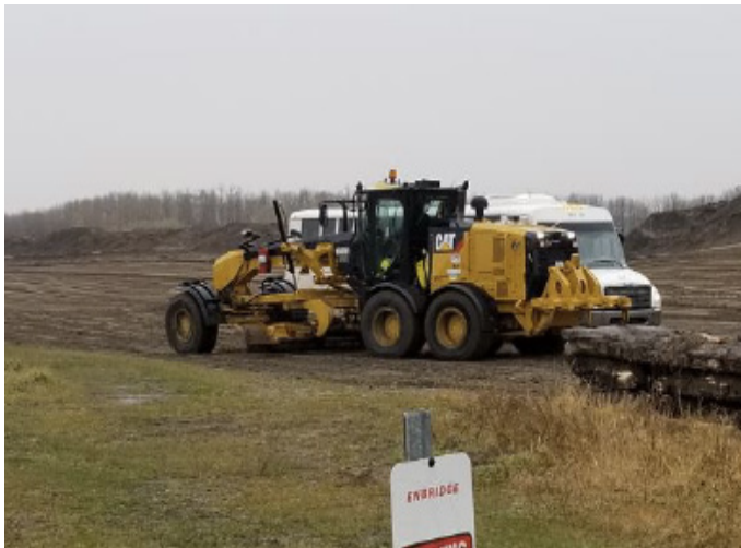
Grader levelling ROW – SF 31 - Oct 12, 2018
